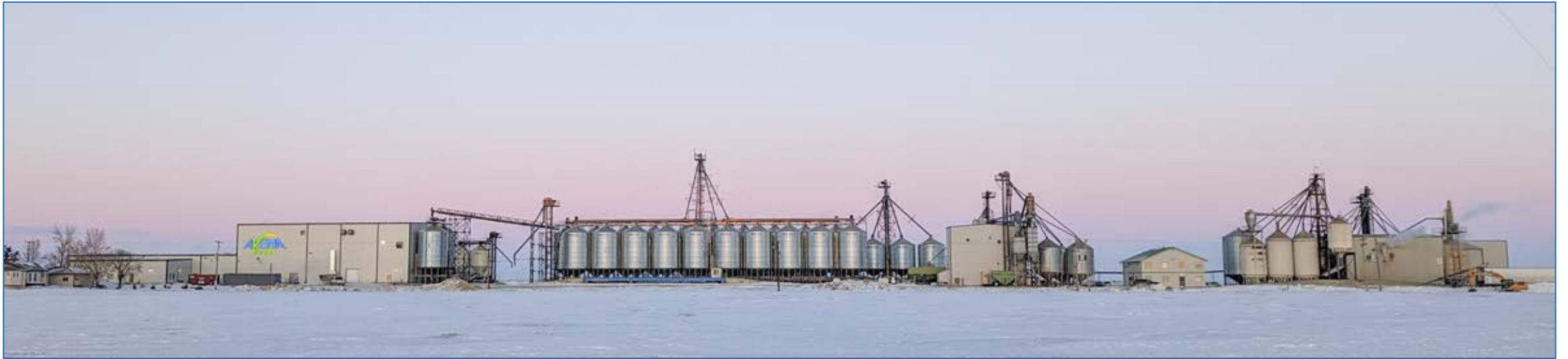
Avena Purity Protocol Oat Mill, Oat Cleaning Plant, Pulse Cleaning Plant, Pea Splitter Rowatt, Saskatchewan
