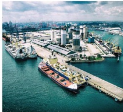
PHOTOGRAPH 20. SOUTHERN PRECINCT CHARACTER
